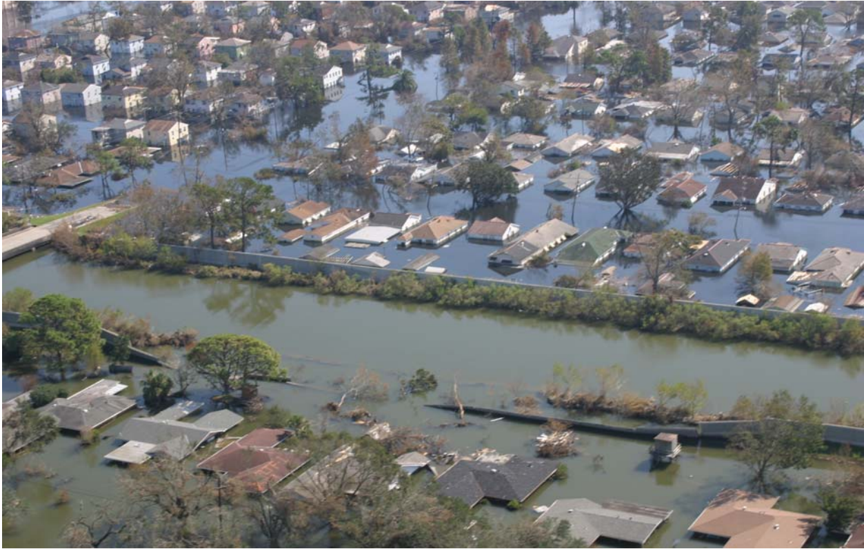
Figure 16. Example of I-wall breach on London Avenue Outfall Canal (north breach) resulting from formation of a crack along the water side of the floodwall, introducing high pore pressures under the levee and causing uplift and failure
