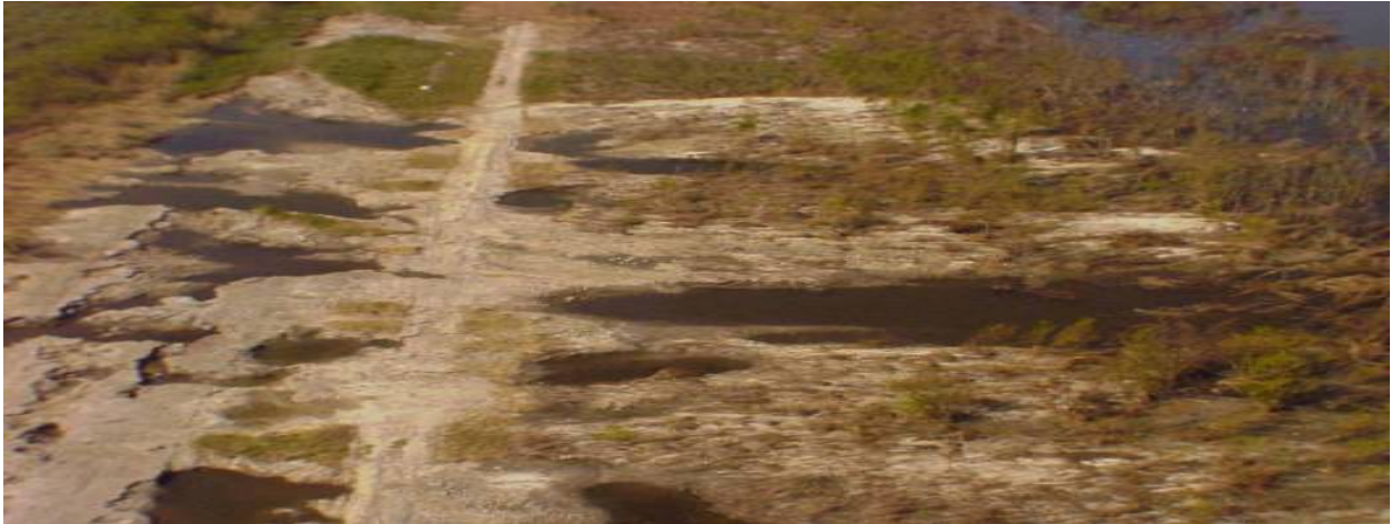
Figure 13. Example of levee along New Orleans East, GIWW, breaching from overtopping and scour of erodible materials
