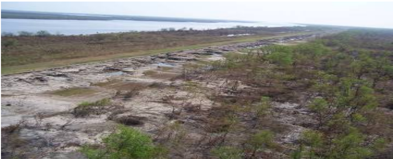
Figure 14. Example of levee breach along MRGO from overtopping and scour of erodible materials
