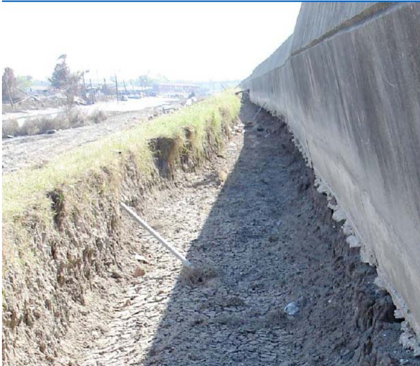
Figure 18. Example of breach along IHNC (east side) from overtopping and scour (top) and scour behind adjacent section that did not fail (bottom)
